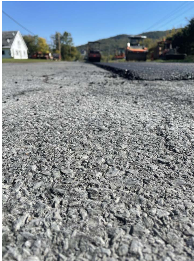
*County Forces Paving County Route 7A - Dresden
